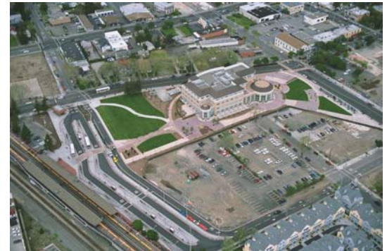
Hayward City Hall and BART Intermodal Transfer Station
