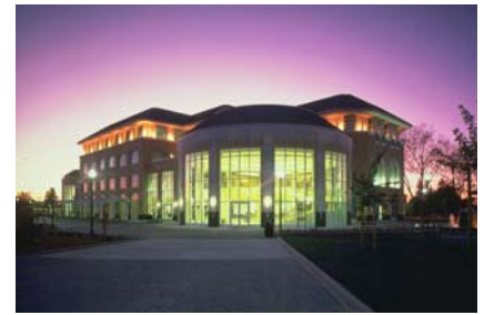
Hayward City Hall (Fully base-isolated with a subterranean garage)
